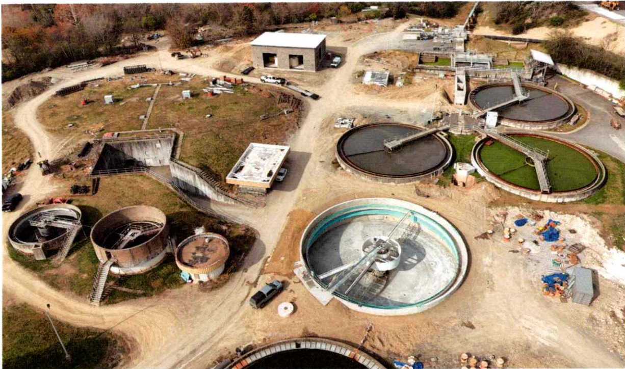
Davidson Drive WWTreatment Plant Clarifier under construction
