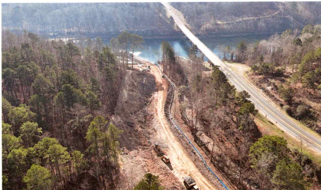
Davidson Drive WWTP Outfall Construction
