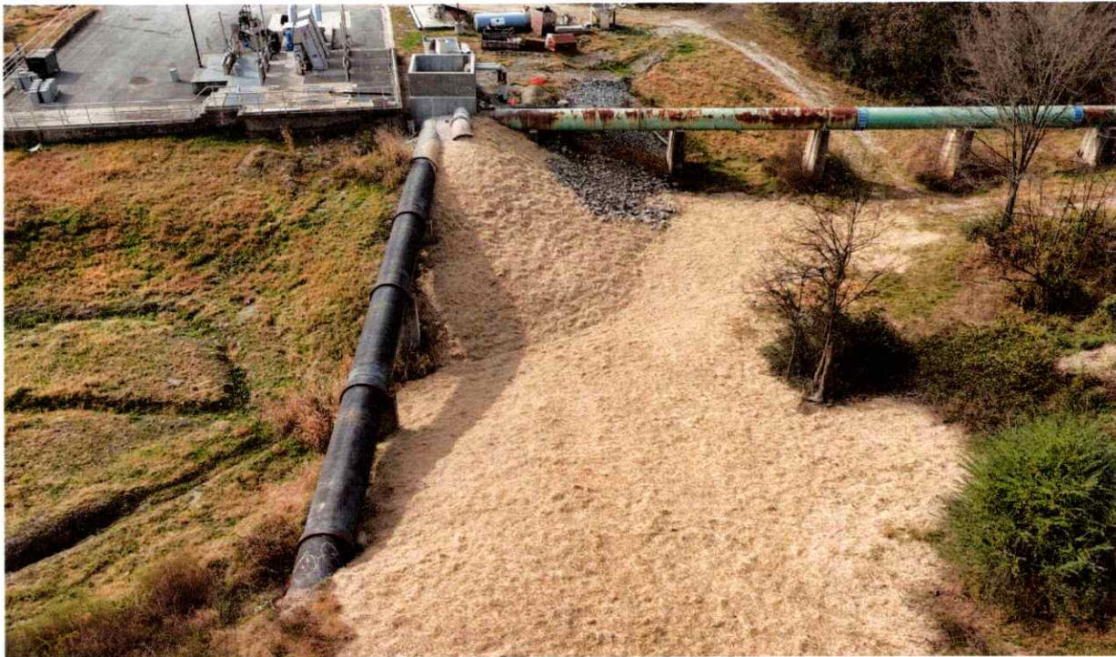
Davidson Drive WWTreatment Plant – End of Force Main from Gulpha Pump Station
