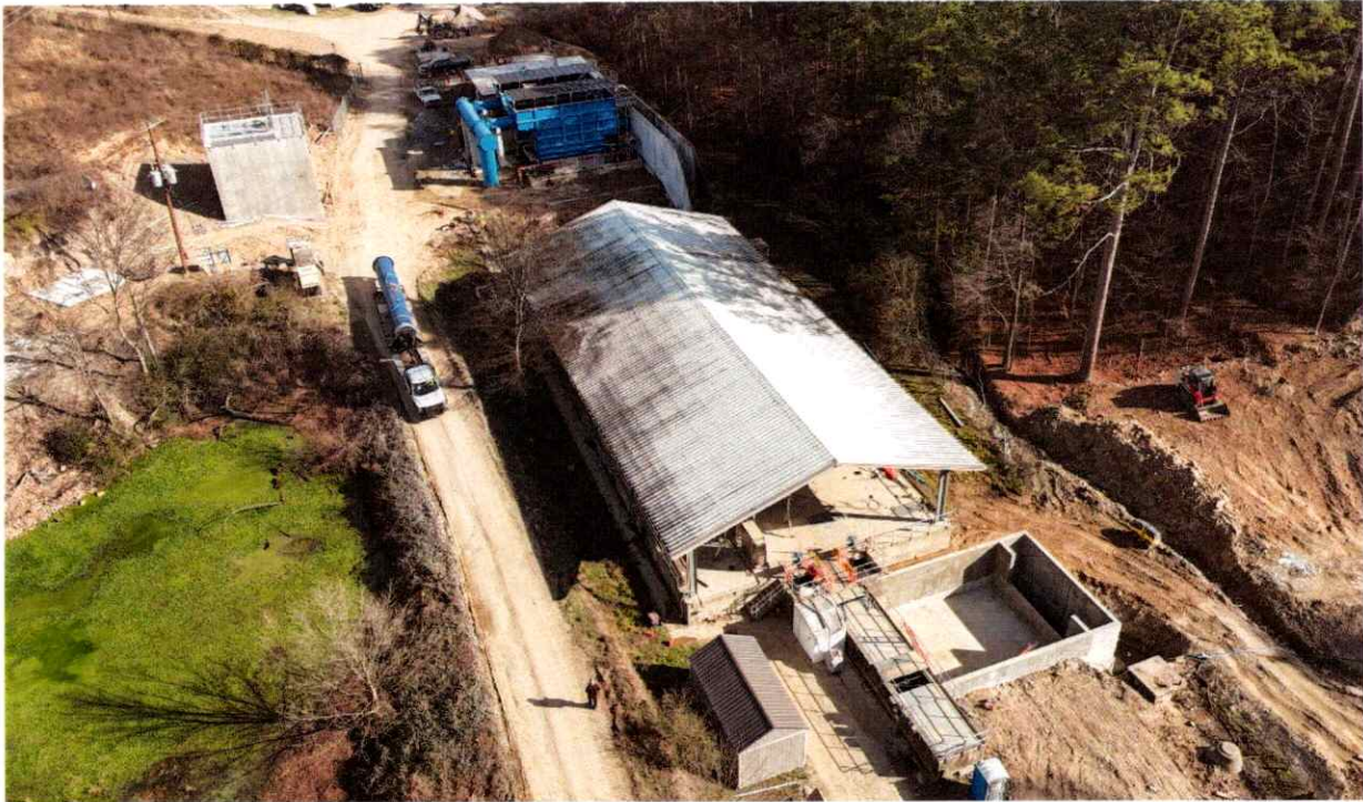
Davidson Drive WWTP Outfall Construction
