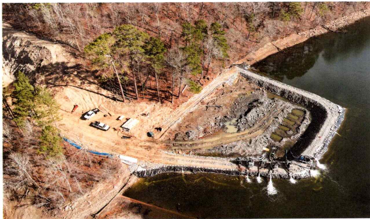
Davidson Drive WWTP Outfall Construction
