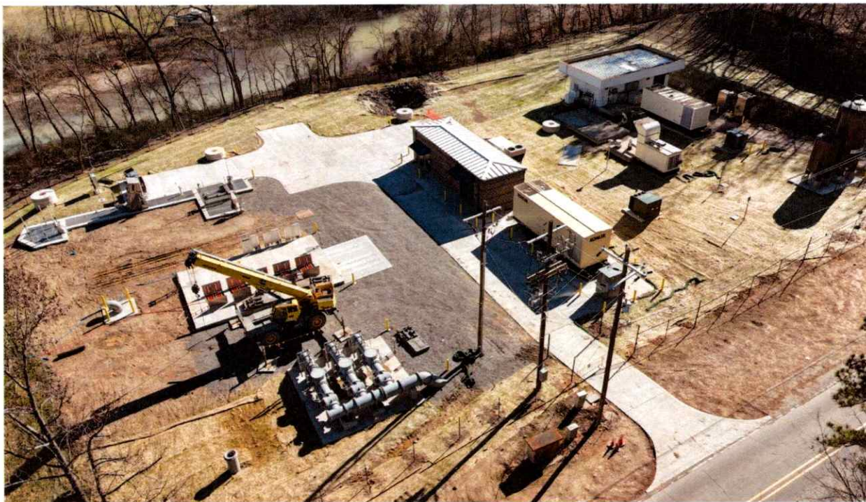
Gulpha Pump Station Construction
