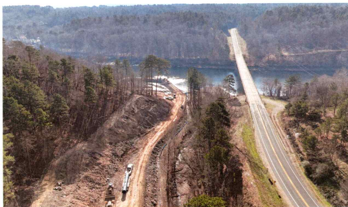
Davidson Drive WWTP Outfall Construction
